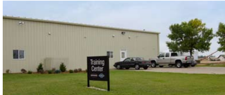
Employee/Customer Training Center
